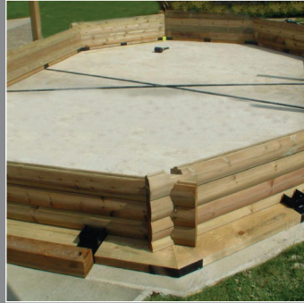
Lay out the base structure and start to build the wooden sections which fit together perfectly
