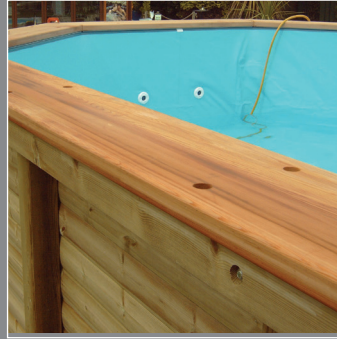
When constructed, add in the liner and fill with water
