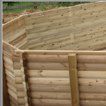
Build the wooden surround
