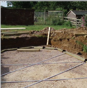
Dig the hole and prepare a flat base
