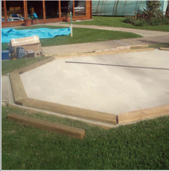
Concrete level base
