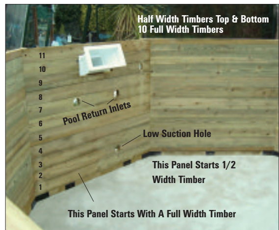
STEP 16 - Where the skimmer is located on a corner wall the low suction is sited at 2.5 log and the returns are positioned at 5.5 log. The skimmer is 9.5 - 10.5 logs. See appendix A / B
