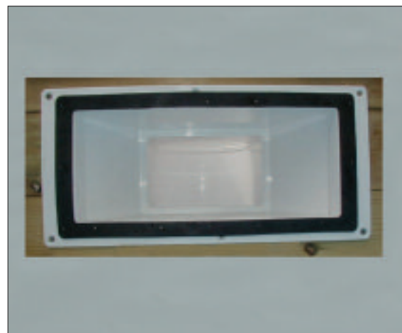
STEP 48 - Cut the foam 20mm clear and around the skimmer face and stick the black seal to skimmer face.
