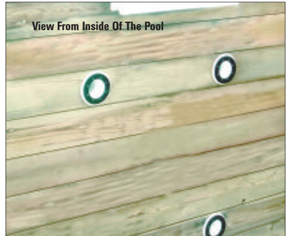
STEP 20 - Fit the return inlet and the lower suction fittings.
