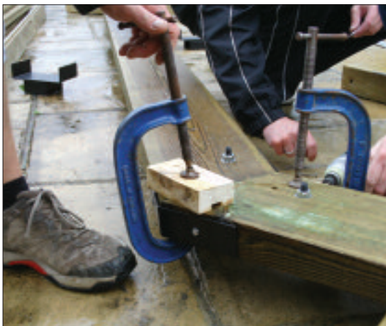
STEP 3 - Use G clamps as shown to aid fitting.
