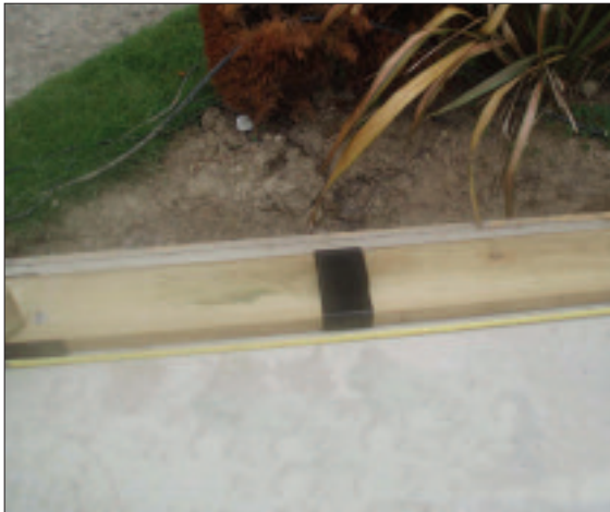
STEP 7 - Position the remaining shoes at the centre of the short base timbers as shown. Do not fix at this stage.
