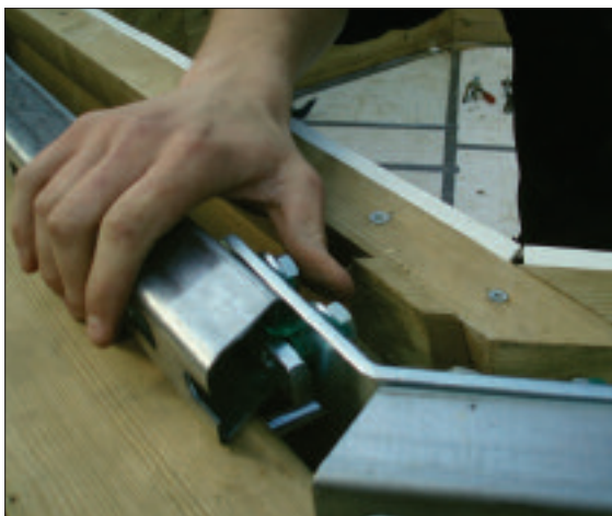
STEP 35 - Insert bracket into next length of steel. Push up to meet the corner and tighten the bolts with the 17mm spanner.
