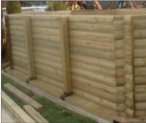
STEP 25 - Place the upright posts in the steel shoes with the holes facing outwards. Do not fix the uprights in the shoes at this stage.
