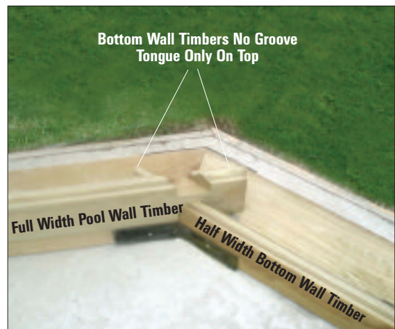
STEP 10 - Line up the inside edge of base timber with the first row of pool wall timbers.
