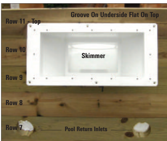
STEP 17 - Insert row 11 with the groove on the underside and the flat on the top.
