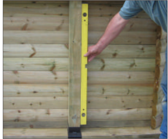
STEP 38 - Check that all the posts are upright. Tap the base left or right as necessary using the mallet.
