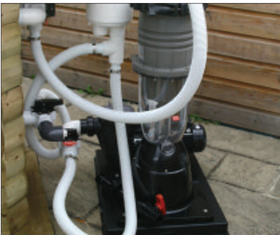
STEP 41 - Assemble the filter and pumps onto the base following the separate instruction which come with the filter.
