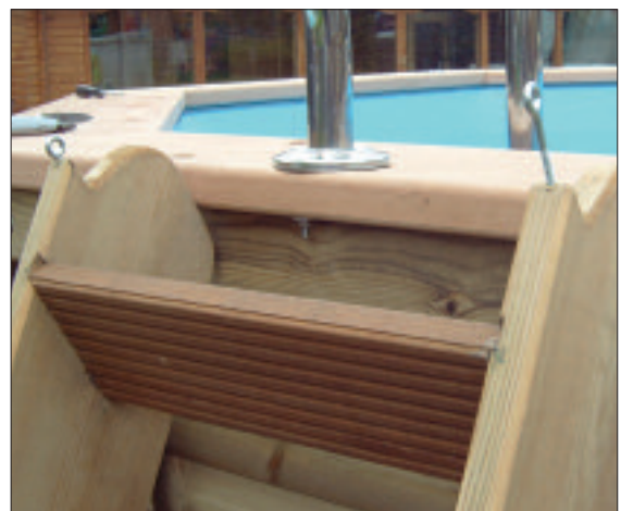
STEP 70 - Screw in the two eye screws into the top of the underside of the wooden pool steps as shown above.
