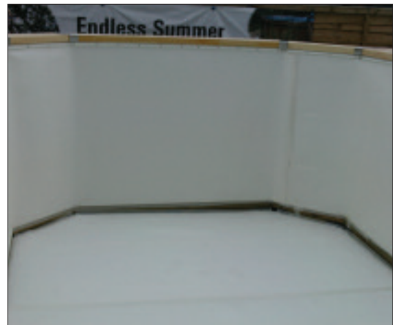
STEP 50 - Completed foam barrier
