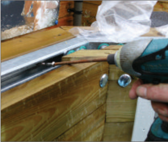
STEP 37 - Screw the metal ring beam to the wooden ring beam using No12 x 2.5 screws SPGP38 and washers SPGP39.
