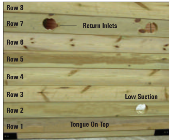
STEP 14 - When preparing the pool please remember to place the timbers so that the return inlets are on row 7 and the low suction point is on row 3.
