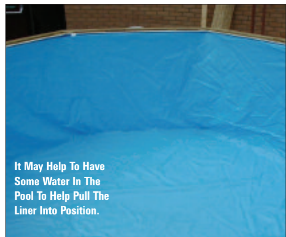
STEP 54 - Continue pushing the liner into the liner-lock all around the pool and then push out the creases with your feet. Do Not wear shoes for this procedure.
