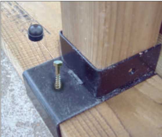
STEP 39 - Fix steel shoe to the base with 10mm coach screws and fit the plastic cap. Do not fix the post to the base shoe at this stage.
