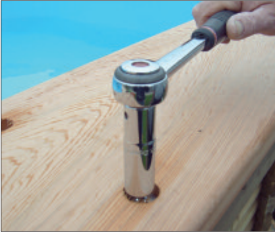
STEP 65 - Insert the 10mm coach screws and washers and gently tighten down with the socket wrench. Repeat around the pool. Once complete fit the chrome caps.
