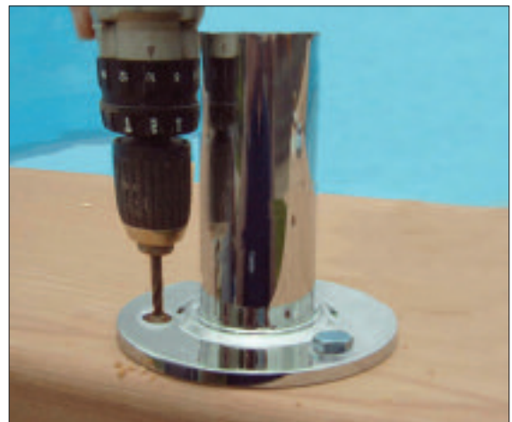
STEP 68 - Drill 6mm pilot holes through the timber. Tighten down with M10 x 100mm coach screws.
