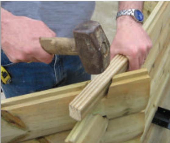
STEP 13 - Tap the timbers down gently using a scrap piece of wood. Line up the tongues and the grooves before tapping.
