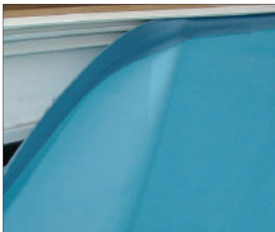
STEP 53 - Push the top of the liner into the top groove of the liner-lock.
