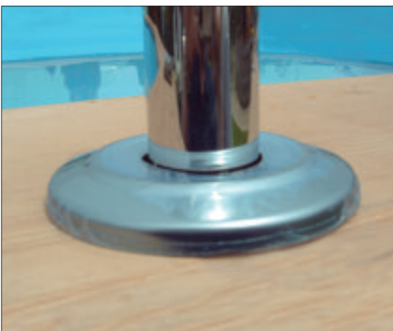
STEP 69 - Place the stainless steel covers and then assemble and fit the steps. Assembly instructions for the steps are in the steps box.
