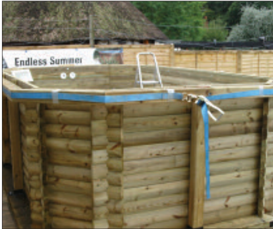
STEP 31 - Using straps around the ring beam whilst fitting makes the job easier.
