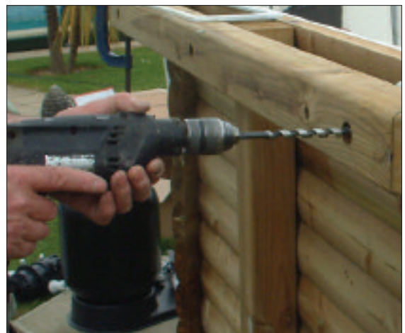
STEP 30 - Drill holes through the timber and pool wall and insert a 230mm x 12mm bolt through from the inside as shown.
