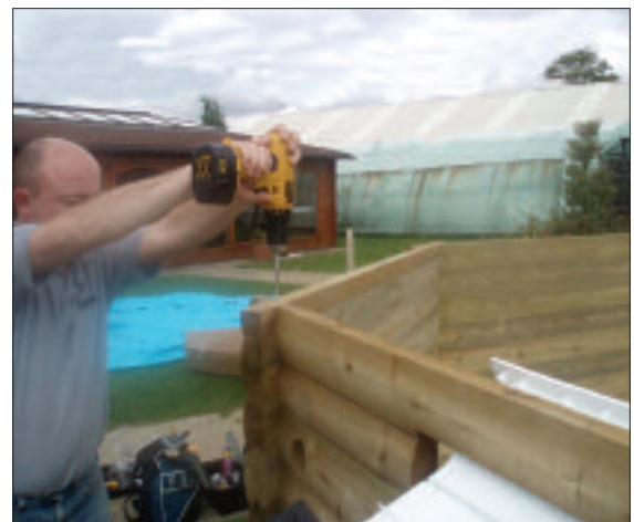
STEP 24 - Repeat on other 3 sides with half timber tops.
