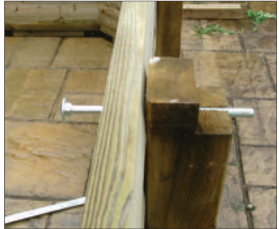
STEP 26 - Align the upright posts with the wall holes.
