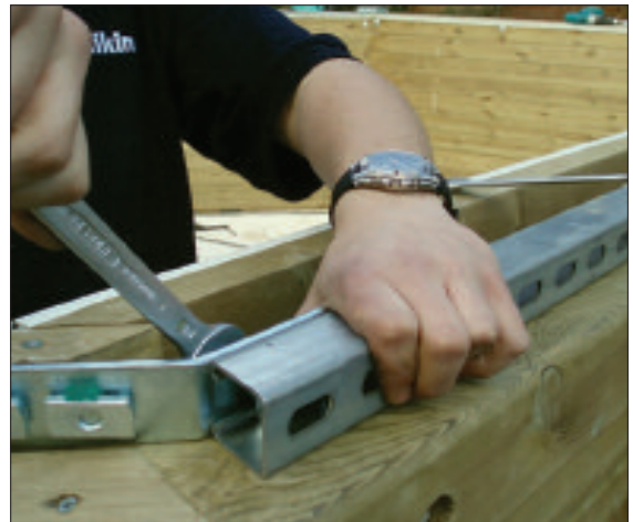
STEP 34 - Lay out the steel inner ring beam round the pool top. Fit the corner connecting brackets to one side of each length. Tighten bolts using 17mm spanner.
