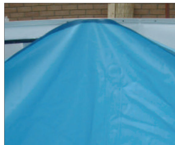
STEP 52 - Start placing the liner in the top groove of the plastic liner-lock. Start from a corner and work your way round.
