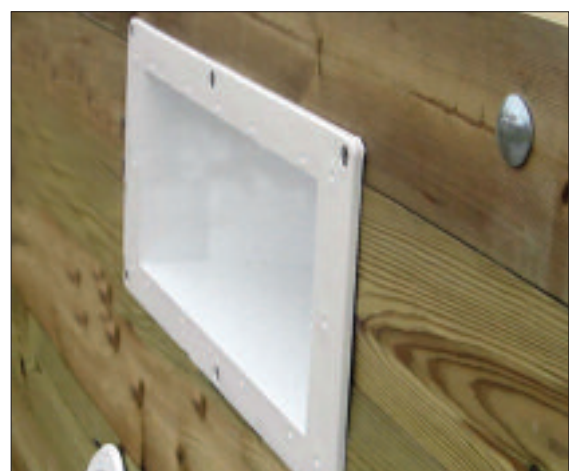
STEP 18 - Fit the skimmer to the pool wall with the 6 No10 x 1" screws provided.
