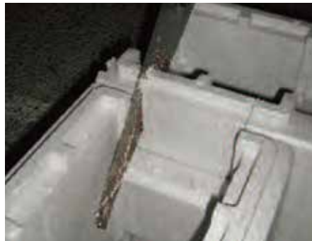
Saw the 1st block from the top and bottom corners (leaving space for concrete + irons). Repeat this cut at each angle and for all levels.
