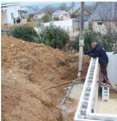
Be careful to prime the pump outside the structure.
