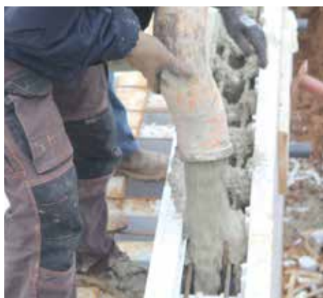
Be careful to prime the pump outside the structure.
