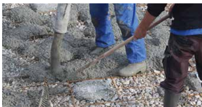
Pouring a flat concrete slab
